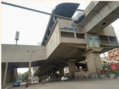
KPHB Metro Station
